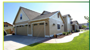
Edgell Building Inc.
